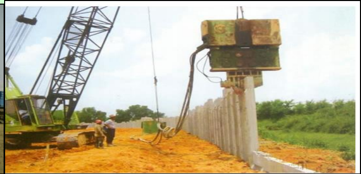
..... Piling Construction works
